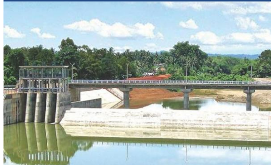
Public access to basic service infrastructure
